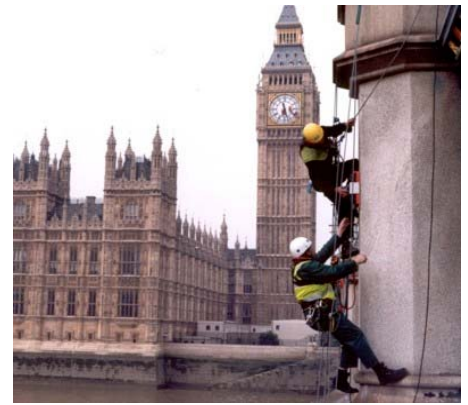
Rope access survey of Westminster Bridge stonework
