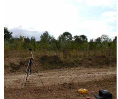
Noise and vibration impact monitoring
