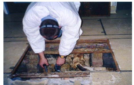
Asbestos surveys and management
