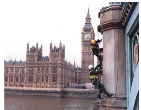
Radar survey of Westminster Bridge
