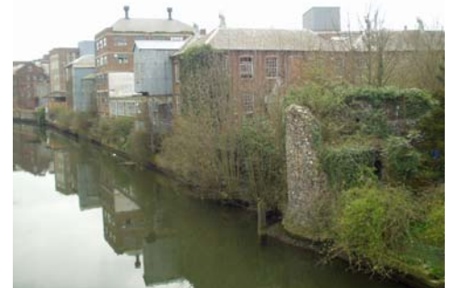
Environmentally sensitive site assessment
