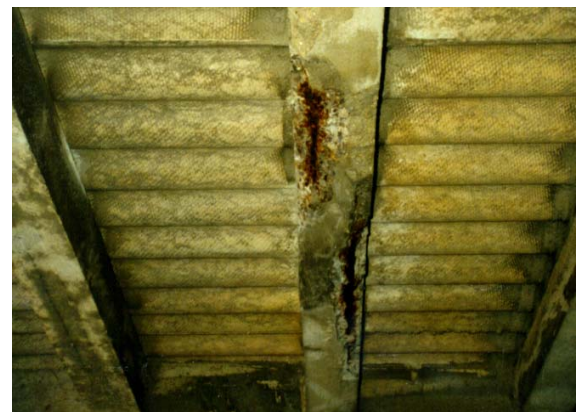
Reinforcement corrosion in a car park
