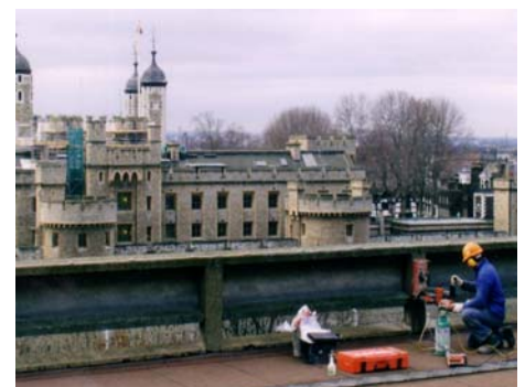
On-site concrete core sampling
