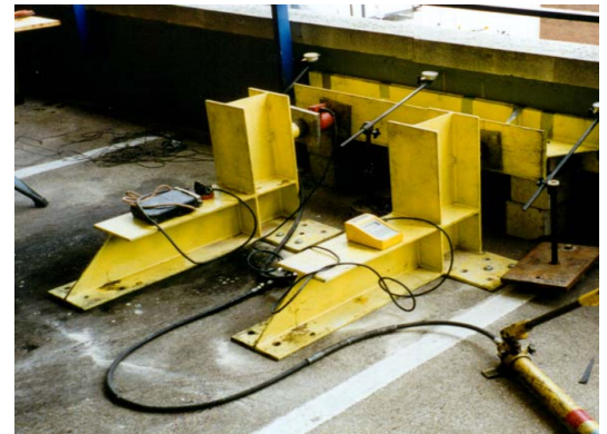
Barrier load testing
