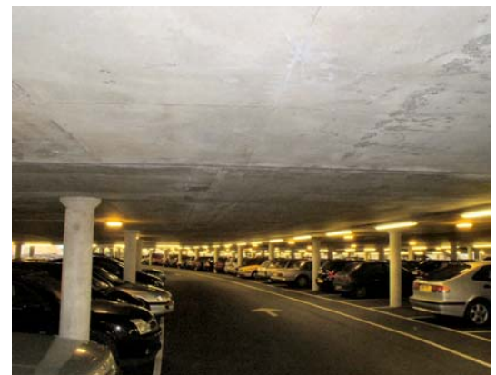
Inspection of concrete structures
